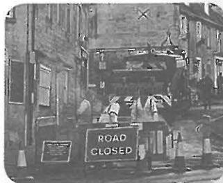
5 Repairs to streets and freeways. (4, 4)
